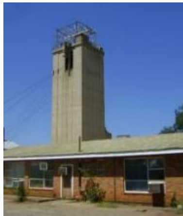
Concrete Headgear of the No.4 Shaft.
