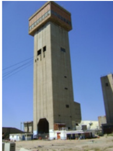
Concrete headgear at the No.1 Shaft.
