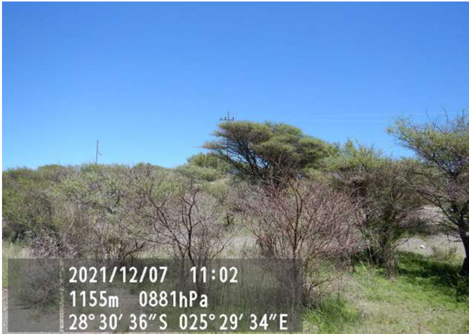
Figure 17: Powerline on top of tailings
