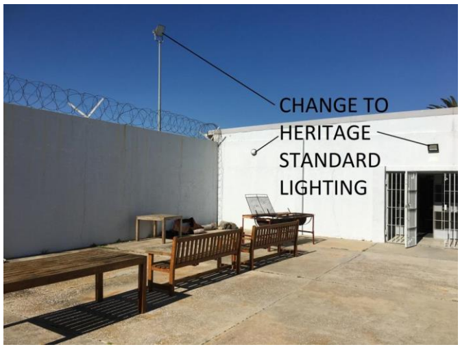
Installation to be corrected
