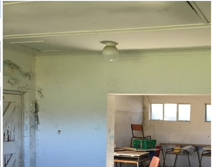
Decide whether to retain cheese fittings or replace with new enclosed LED strip light
