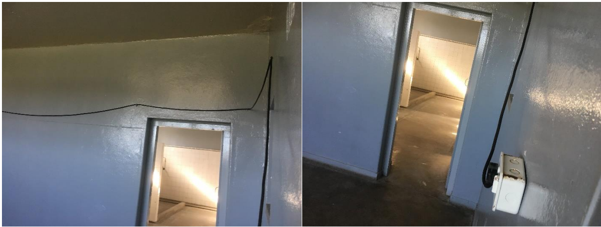
Block F: Remove surface mount cable/extension
