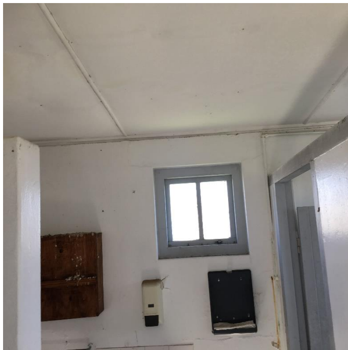
Install new lighting in all ablutions buildings
