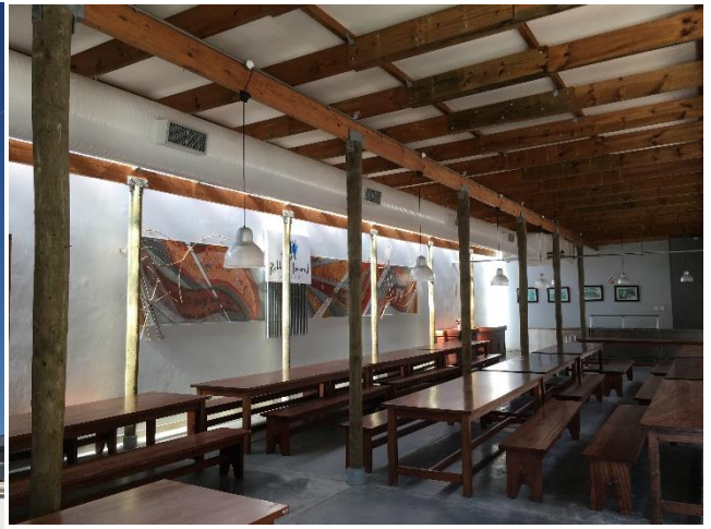
Correct lighting and surface mount conduit to heritage standard if required
