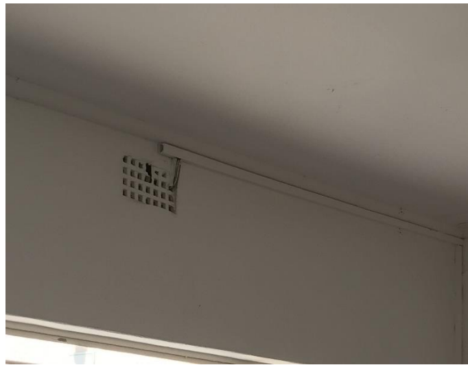
Trunking and wiring to be removed and relocated into ceiling void
