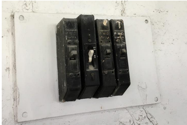
Disconnect & preserve old switchboard & install new DB
