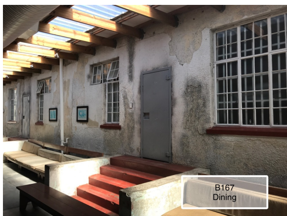
Fig 5. Black mould on walls in dining area. Causes need to be established
