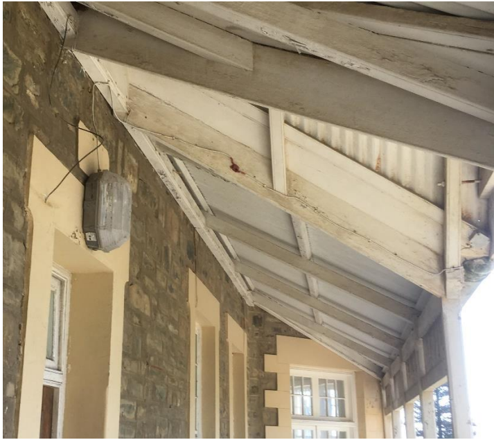
Remove surface wiring and hide away new wiring
