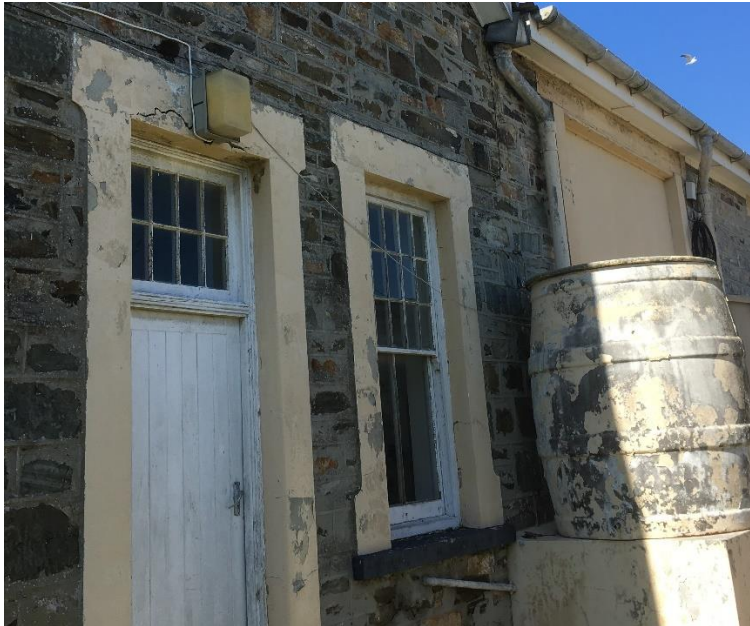
Remove bulkhead and all surface mounted cables
