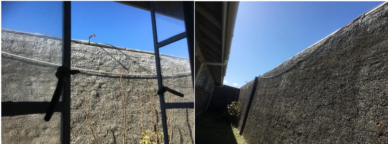
Block F: Remove surface mount cable/extension
