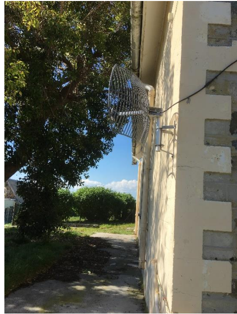
Remove surface mounted fixtures
