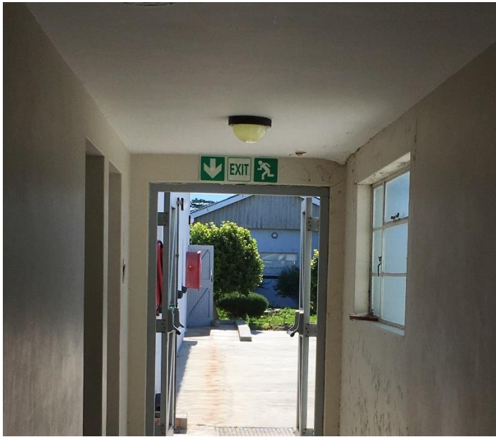
Replace light fitting with heritage standard
