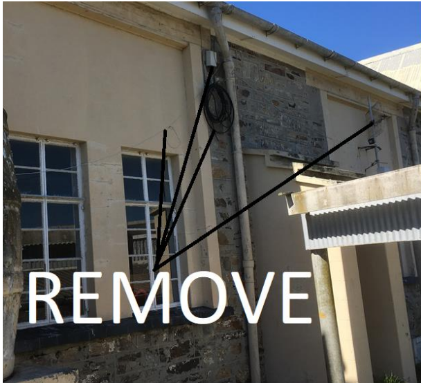
Remove all surface mounted fixtures and cables
