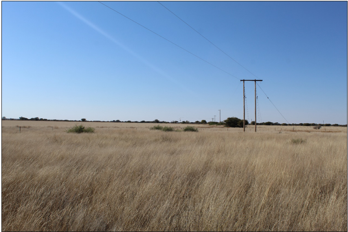
Figure 2: Eastern end of the proposed powerline; the line will run alongside an existing line.
