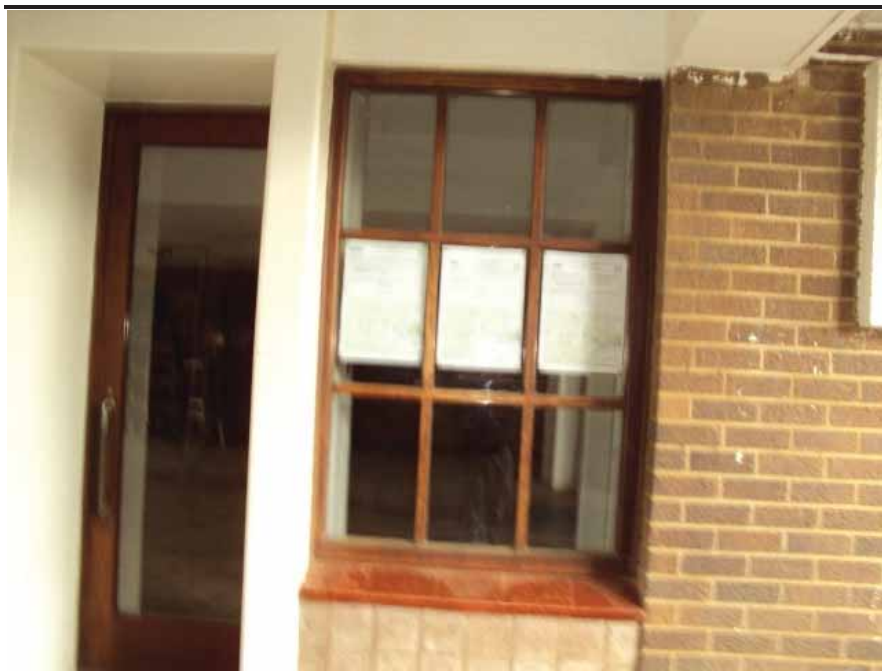
Photo 11 Site Notice Placement - Mkhondo Municipality
