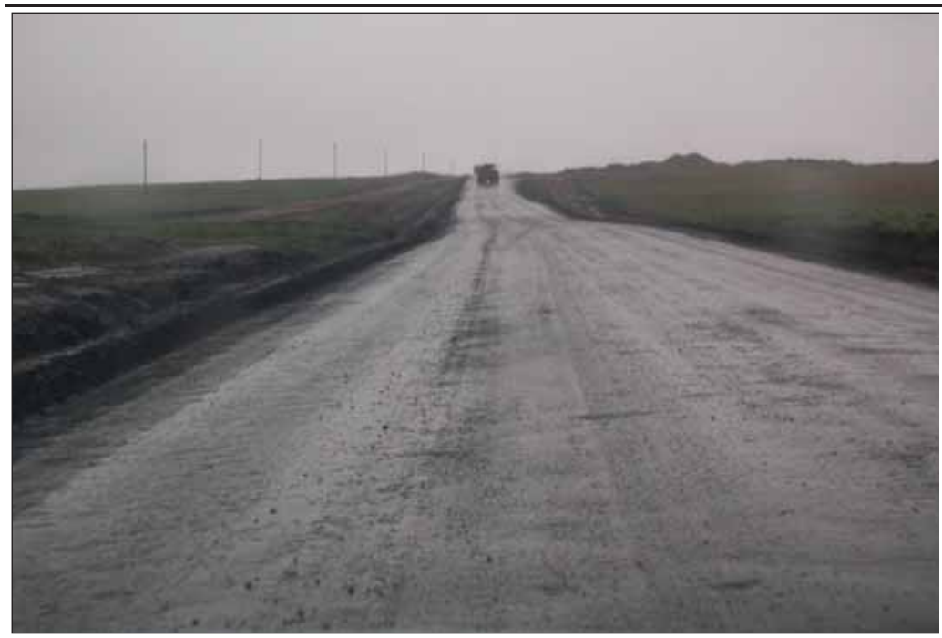
Figure 7.30 Dust Mitigation (Water Spraying) on Public Roads to Panbult Siding
