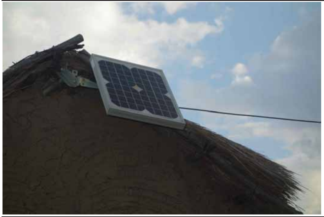
Figure 8.9 Government Provided Solar Panel for Charging Mobile Phones and Batteries
