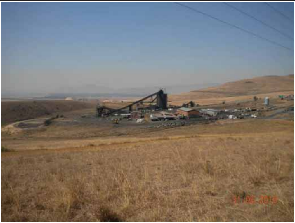
Figure 3.3 Example of the Infrastructure and General Site Layout Associated with a Main Mine Adit
