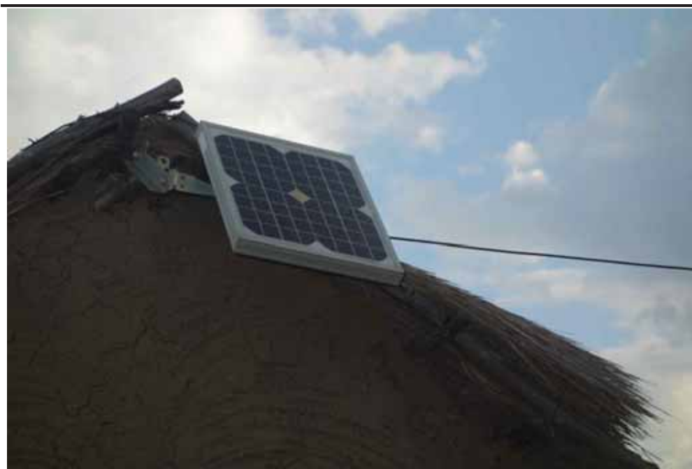
Figure 7.10 Government Provided Solar Panel for Charging Mobile Phones and Batteries
