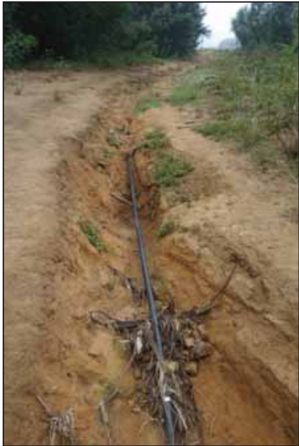
PVC pipes transporting water to homestead tanks and taps (2 above and below left)
