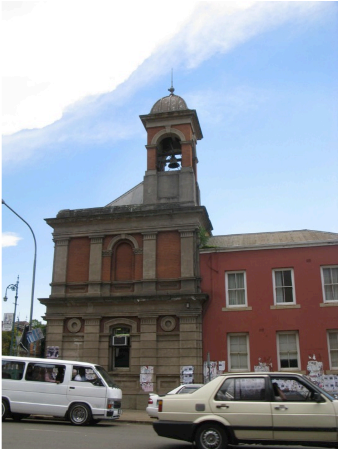
Part south-east corner of Publicity House facing Langalibalele Street
