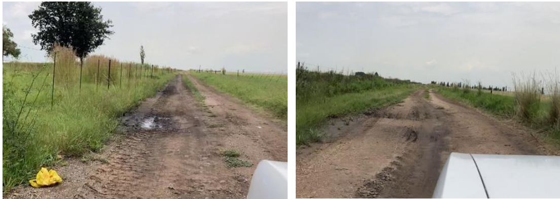
Figure 11-50: Status of the Gravel Road
