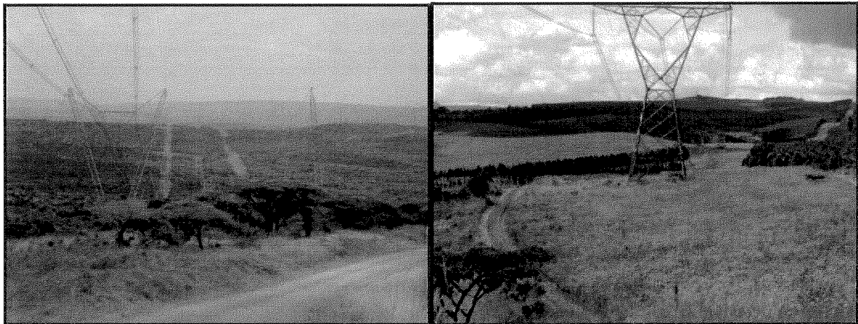
Figure 8-69: View of existing power lines in the study area.
