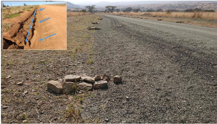
Figure 6-3 Example of road margin erosion prevention
