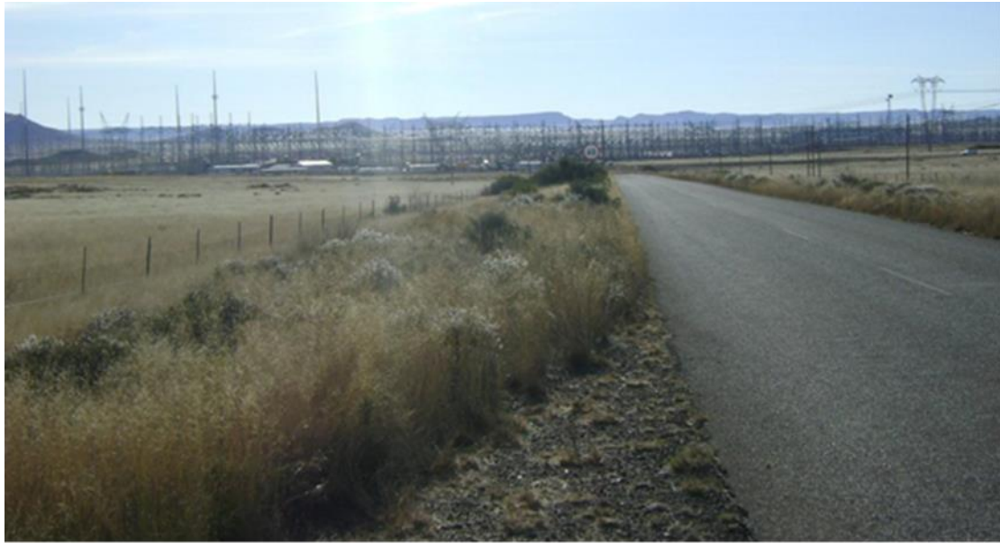
Figure 7: The Hydra Substation in the west of the study area.
