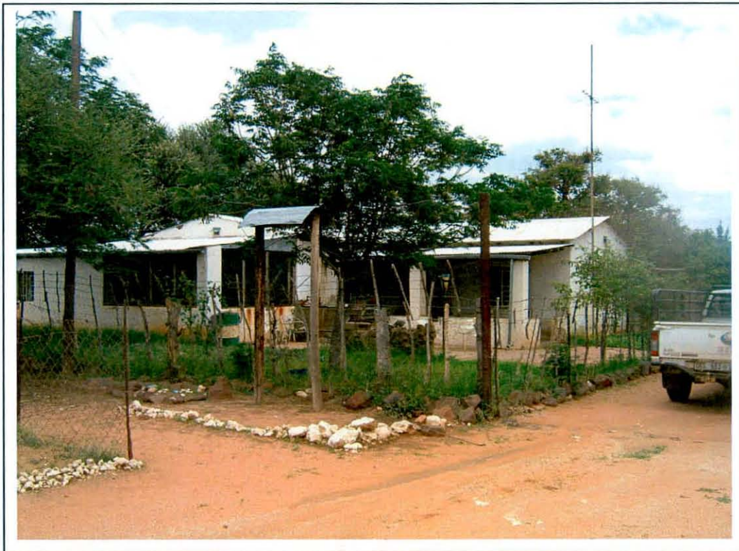
Figure 6- A historical house on Moonlight 111LR. This residence dates from the 1930's or 1940's and was constructed with clay bricks and thereafter white-washed. It is fitted with a pitched corrugated iron roof (above).
