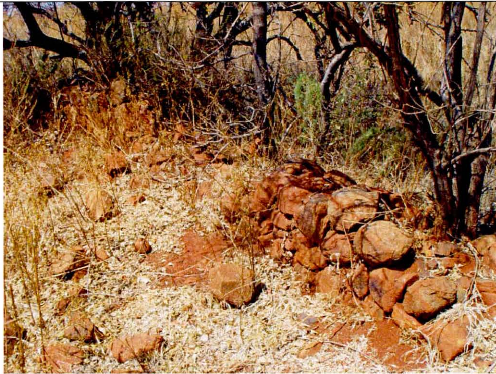
Figure 7: Foundation of structure.
