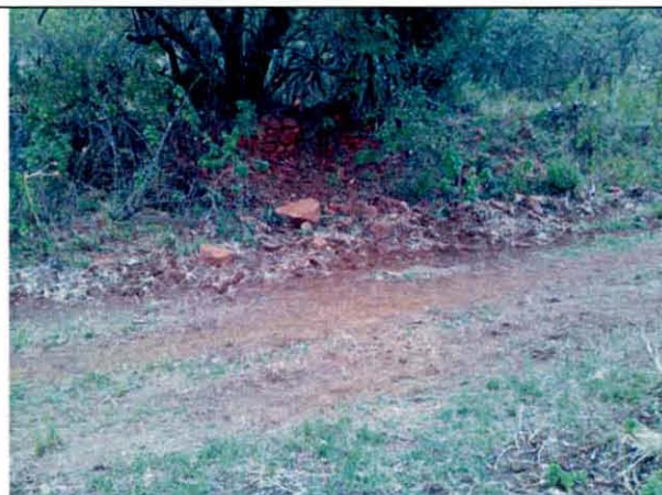
Figure 18: Damage to the site by a new access road
