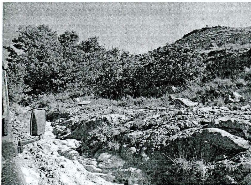
View of the current stormwater measures along the road
