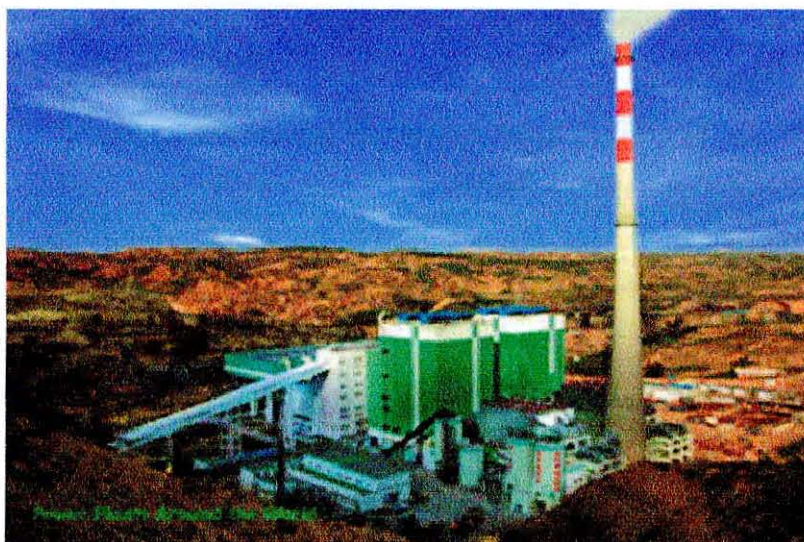
2x135 MW CFB Shendong Baode Power Plant in Shanxi, China (Source: www.industcards.com/st-coal-china-shanxi.htm )
