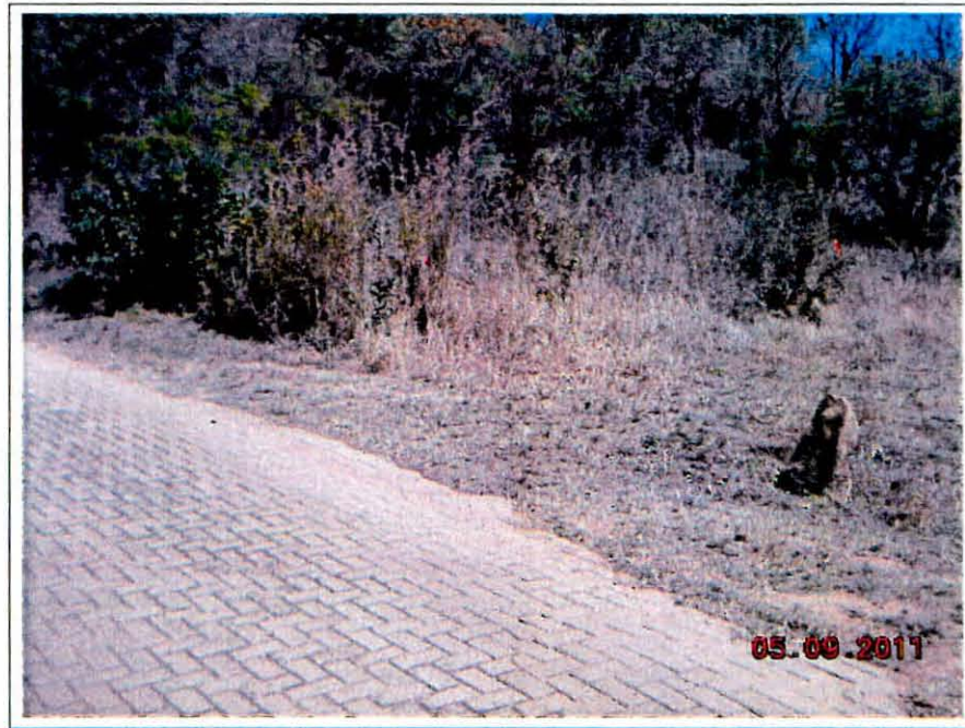
13. General view on site establishment area
