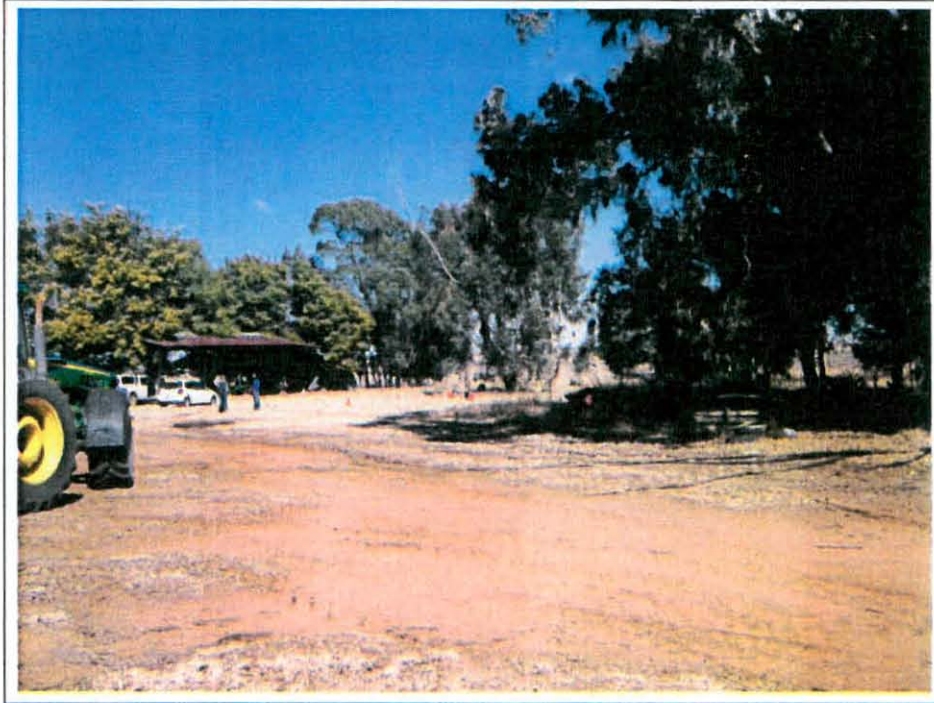
13. General view on site establishment area
