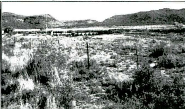
Stormberg River with wetland behind weir
