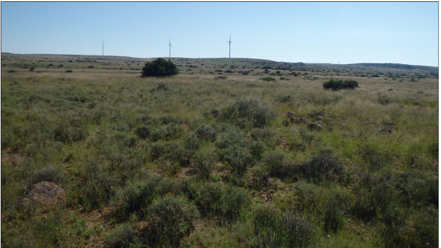
Figure 5.1: Contextual Image of development area - existing turbines from an adjacent project
