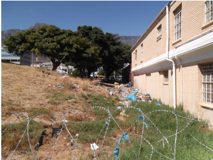
Fig 15 - Building as boundary. Christiaan Barnard St on the left
