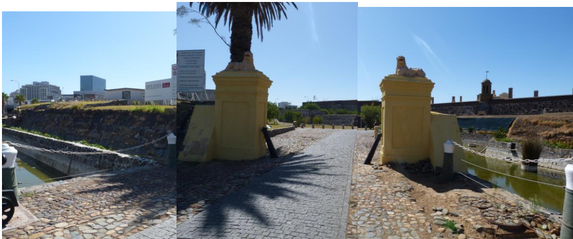
Fig 9 – Existing opening at the Lion Gate
