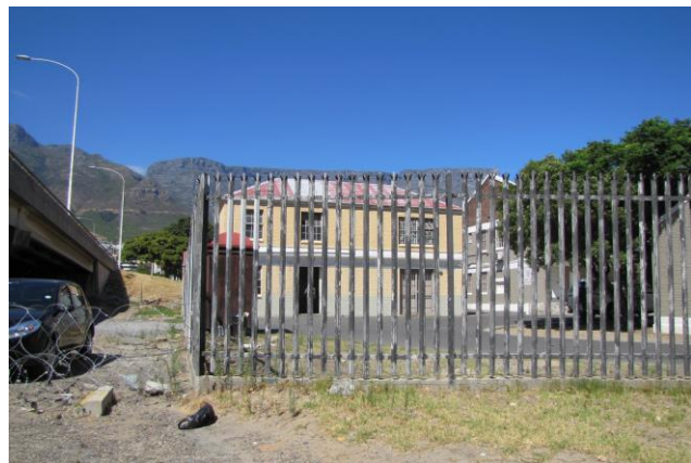
Fig 14 – Contemporary fencing onto which the new will link
