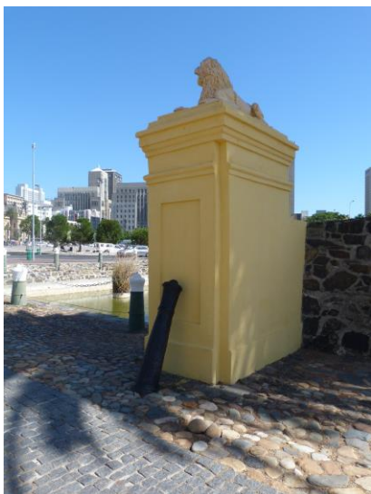
Fig 10 - Existing recess for gate
