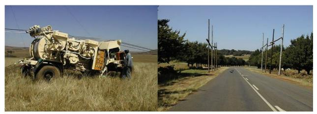
Figure 3.15: Stringing of conductors (power lines) (Step 13)
