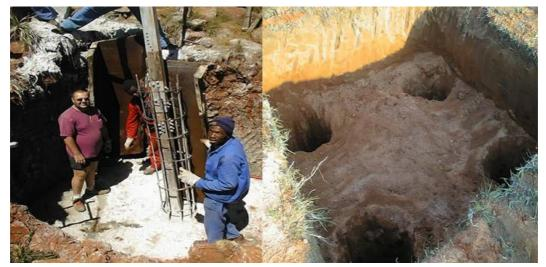
Figure 3.13: Construction of tower foundations (Step 11)
