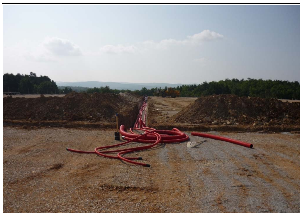
Figure 13.1 Example of Trenching
