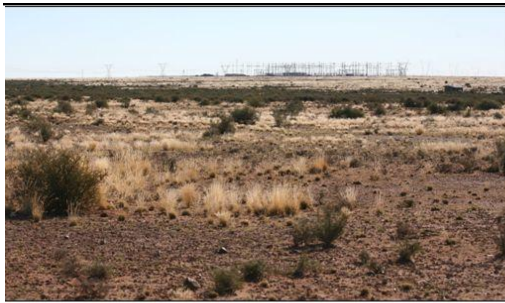
Figure 4.3 Aries Substation in background
