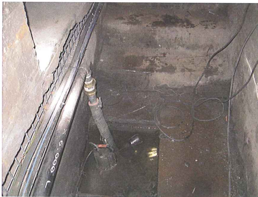
Plate 8-2: Example of surface water monitoring point: Spring water underneath Furnace E
