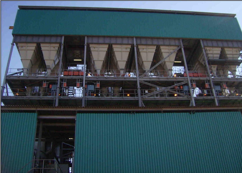
Plate 3.11: Retort feed bins above the retorts.
