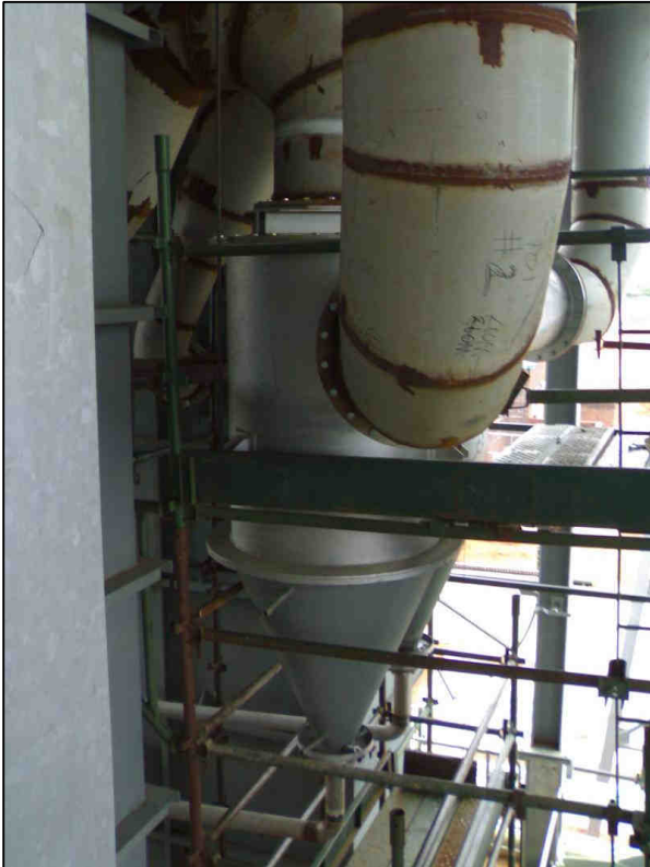
Plate 3.18: The cyclonic separator.
