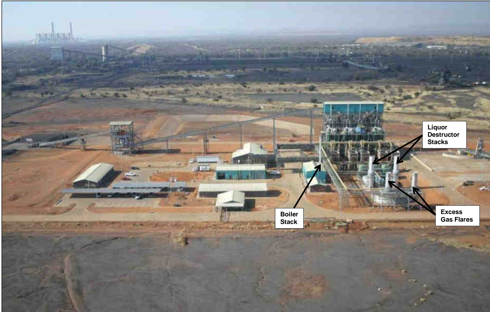
Figure 4.14: Location of Gas Emissions Stacks at the Existing Char Manufacturing Plant.
