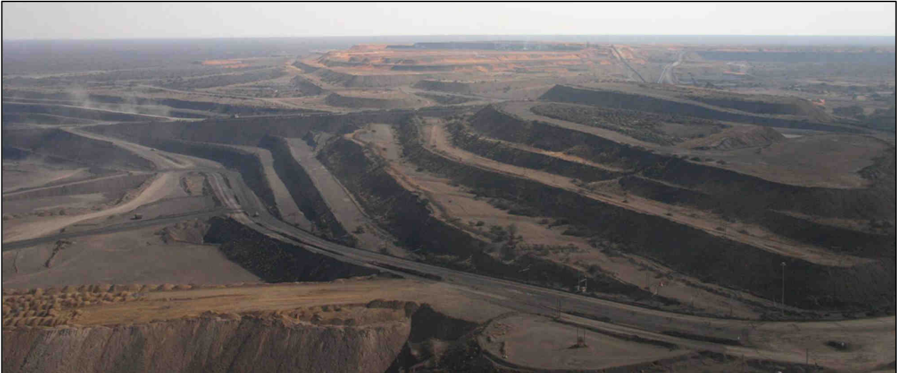
Plate 3.6: Aerial view of the Grootegeluk Coal mine showing the mining benches.
