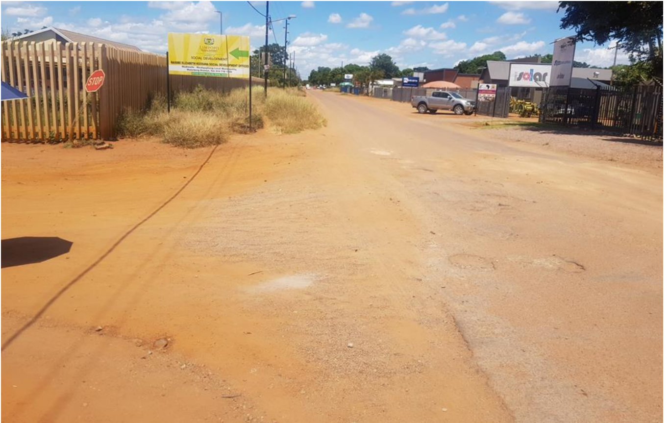
Figure 8 Access road – 1 st street
