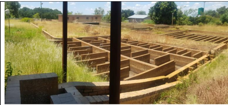
Raw water induced with coagulants and lime is then shocked by letting water run through inlet works prior being conveyed to settlement tank.
