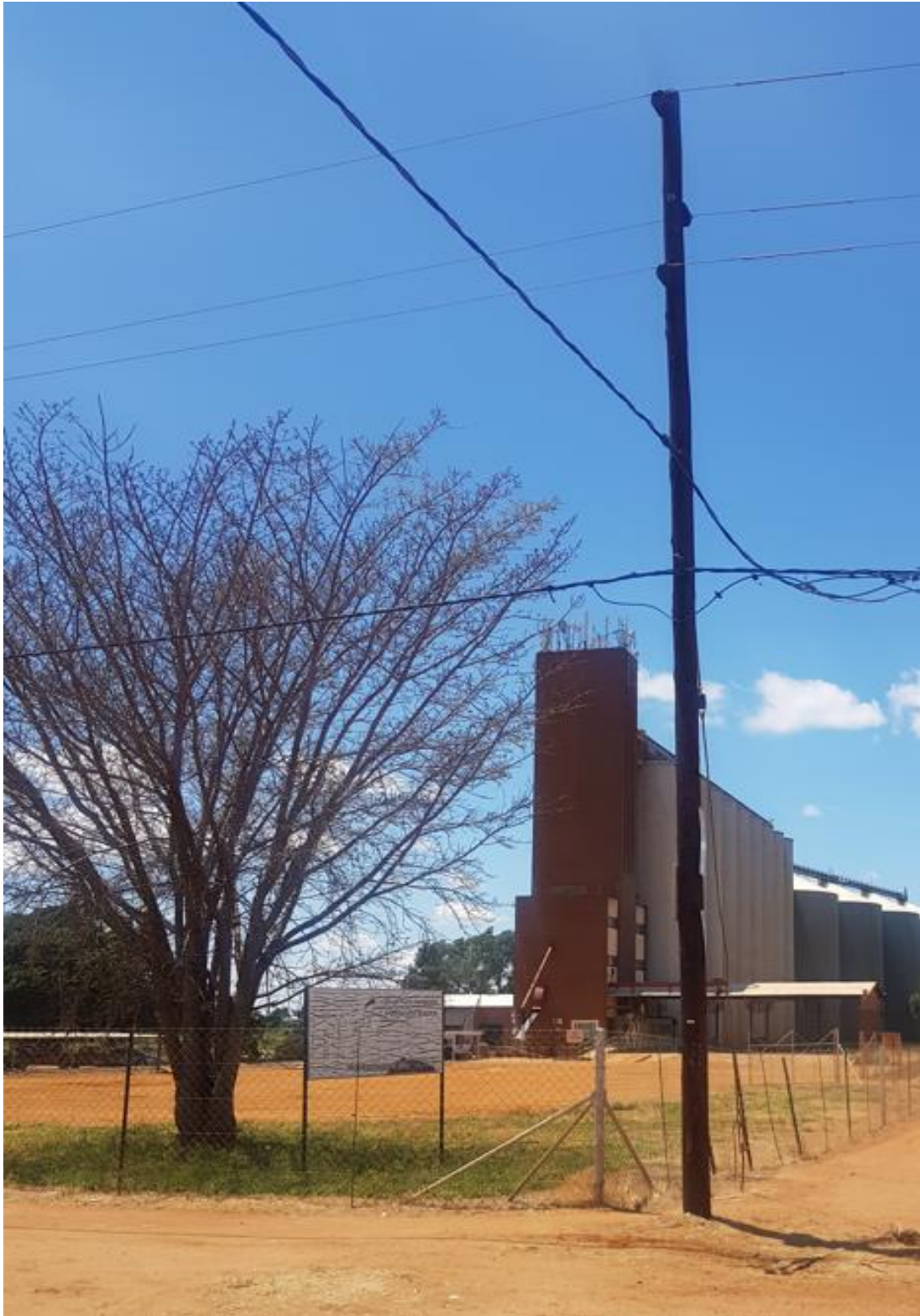
Figure 17 Electrical lines onsite
