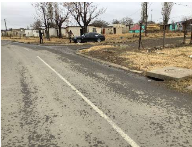
Figure 38: Blocked Kerb inlet on Dr Rolihlahla Drive
