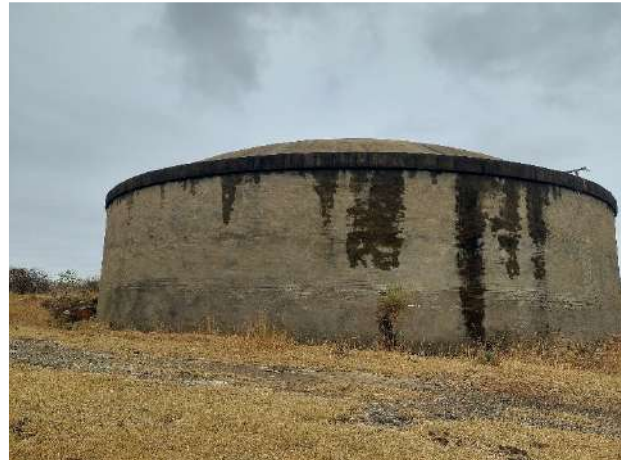
Figure 4: Aasvoelkop Reservoir Two
