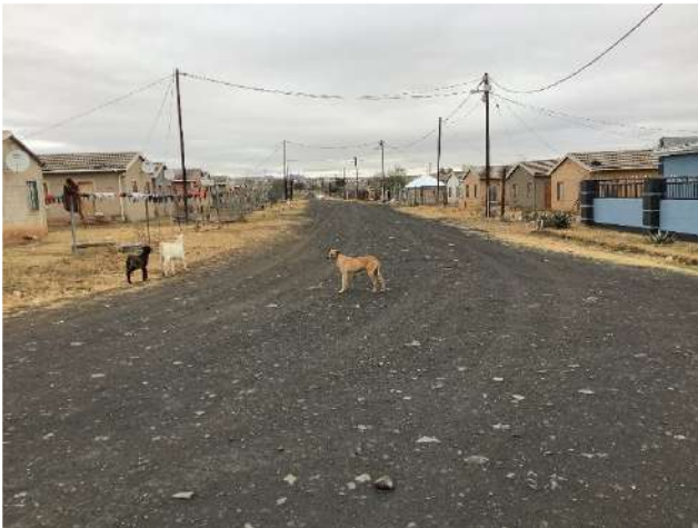
Figure 36: No stormwater was noted on the internal roads
