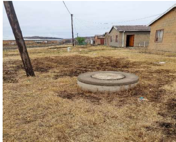
Figure 10: Water Meter in relation to Sewer Manhole
