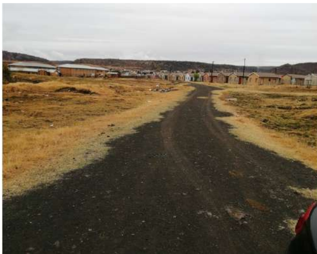
Figure 31: Gravel road Sambane Road
