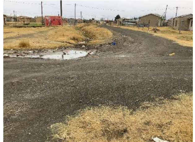
Figure 40: Earth drain blocked
