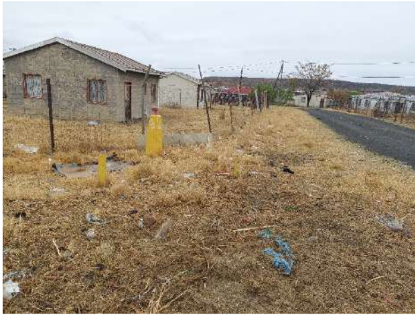
Figure 11: Erf 1926 and Erf 2037 Fire Hydrant
