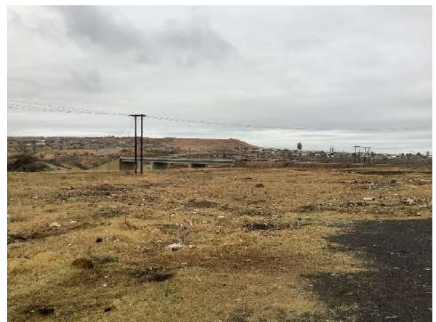
Figure 26: Bridge over Kliprivier
