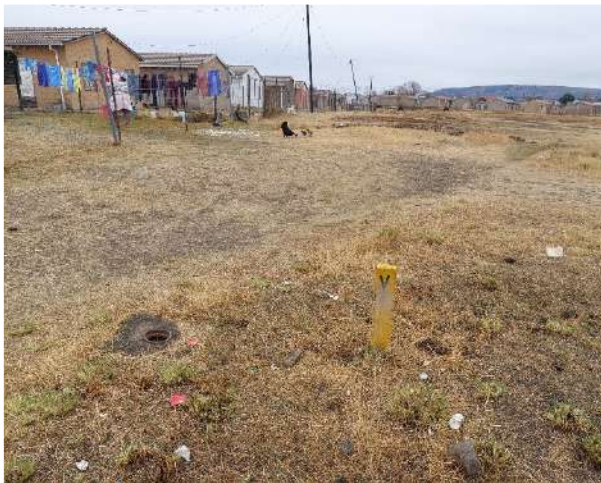
Figure 13: Water Valve and Marker Erf 1916 and 1408
