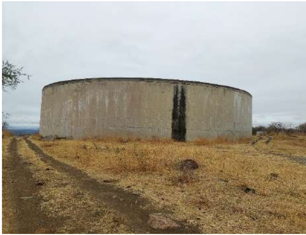
Figure 3: Aasvoelkop Reservoir One
