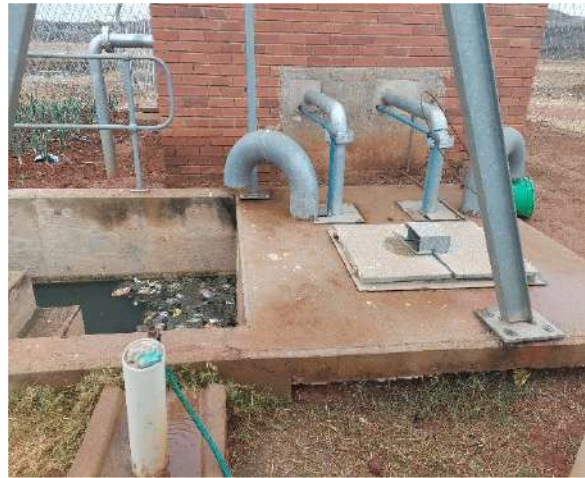
Figure 17: One of Erf 6 Pump Stations
