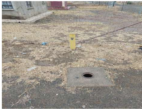
Figure 8: Erf 6 Ezakheni Fire Hydrant Valve
