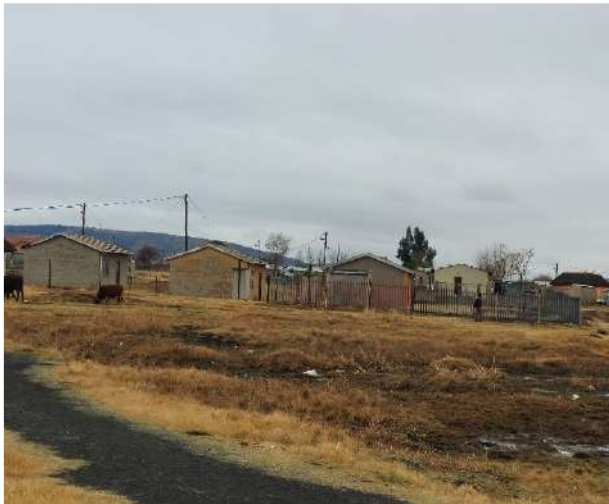
Figure 21: Erf 1912 and Erf 1408 Toilets and Stands
