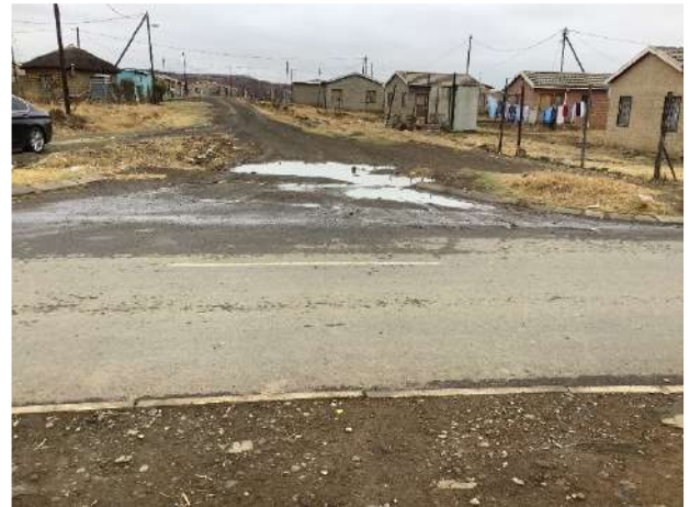
Figure 37: Stormwater ponding on Dr Rolihlahla Drive
