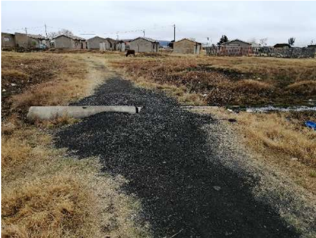
Figure 39: Stormwater pipe from a property into the wetland
