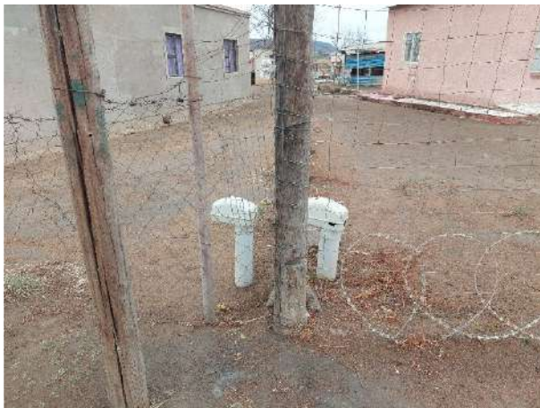
Figure 5: Water Meters in Erf 6 Ezakheni
