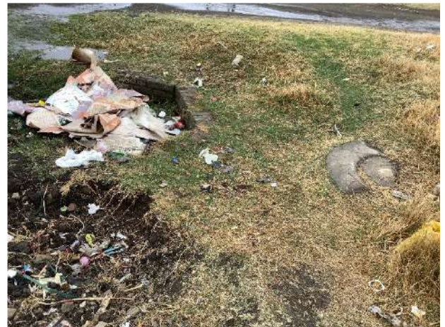
Figure 42: Blocked stormwater outlet on Sigwala Road
