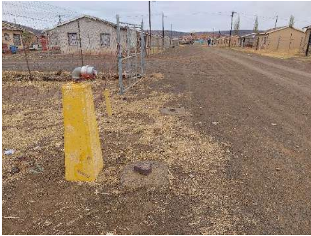
Figure 7: Erf 6 Ezakheni Fire Hydrant
