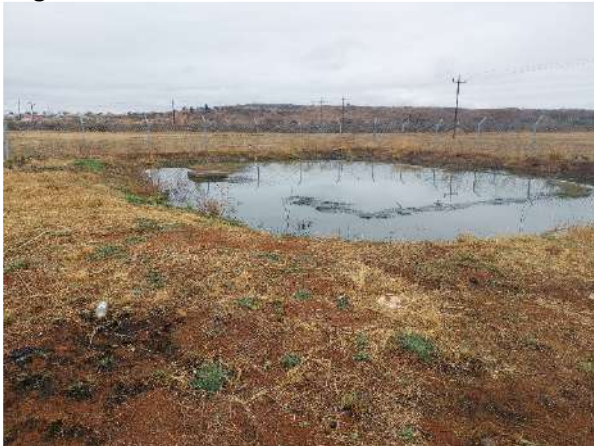
Figure 18: Retention Pond at the Erf 6 pumpstation
