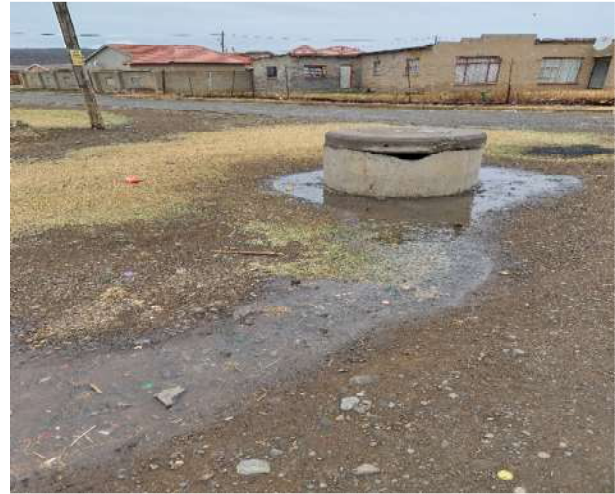
Figure 20: Blocked Sewer Manhole
