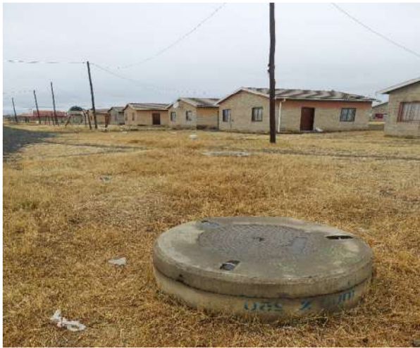
Figure 19: Sewer manholes in Erf 1926 and Erf 2037
