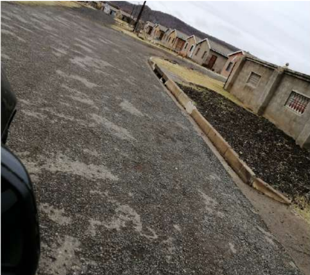
Figure 45: Kerb Inlet in good condition
