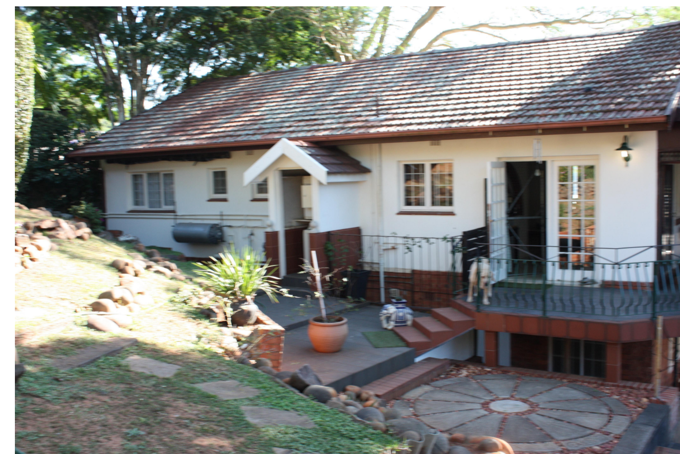
BACKSIDE VIEW FROM BACKYARD
