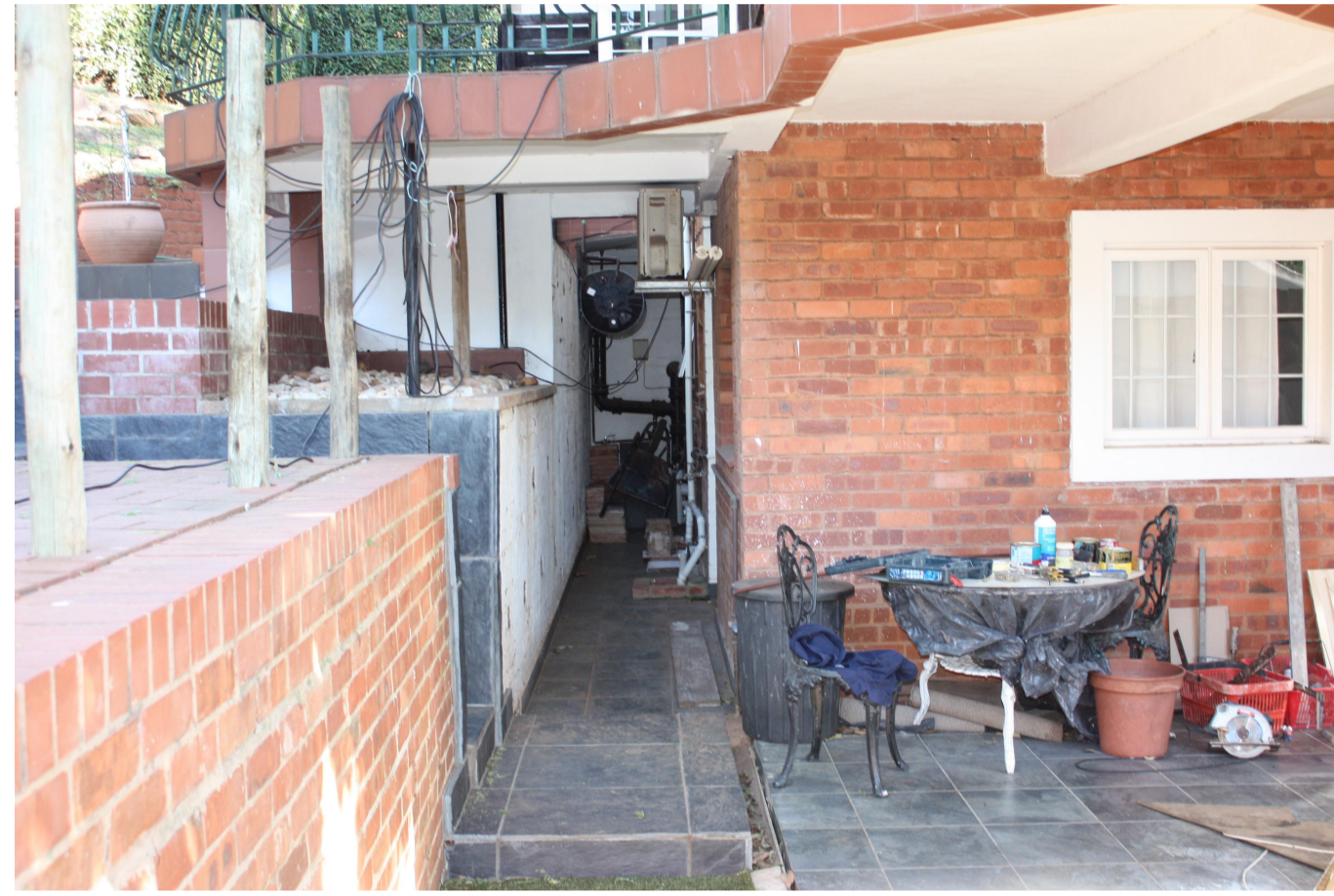
NORTH WESTERN VIEW OF HOUSE
