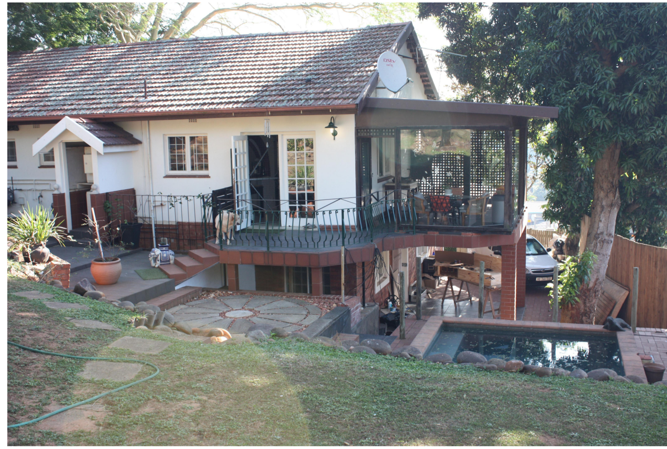
NORTH WESTERN VIEW
