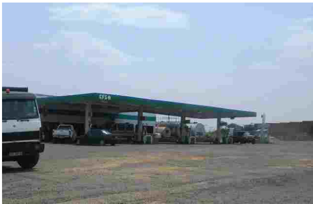
Photo 1: Existing Filling Station on site.
