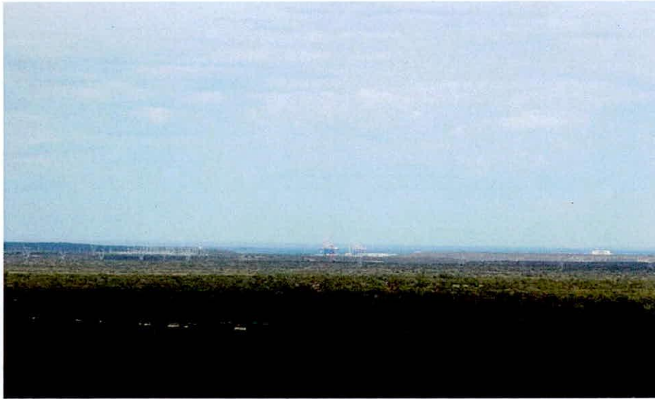
Figure 3.4 Large cranes at Port Ngqura visible from 15km away. The wind turbine will also be in this view and will be comparable in size.
