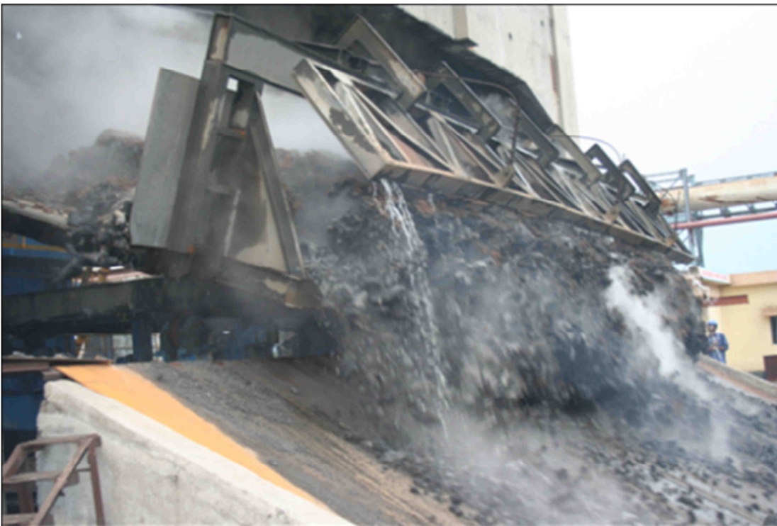
Figure 2.11: Discharging quenched coke on to a coke wharf (similar to proposed Market Coke Plant) (Courtesy Sinosteel).
