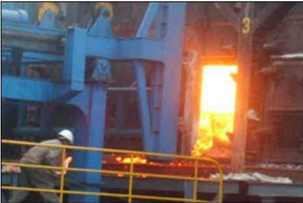
Figure 2.8: Pushing/charging machine opening coke oven door. View of heated coke cake in oven (Courtesy Sinosteel)
