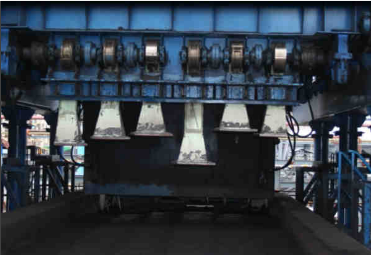
Figure 2.3: Coal cake being compressed by stamping machine (Courtesy Sinosteel)
