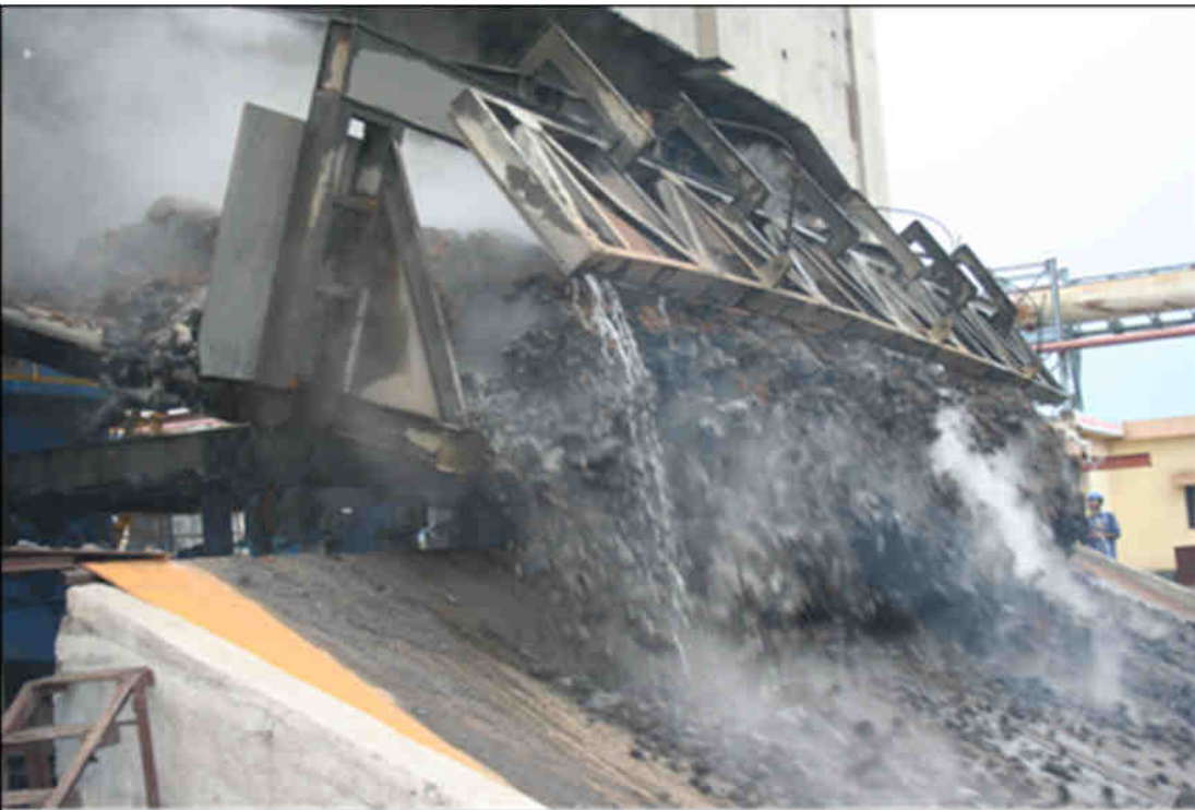
Figure 3.14: Discharging quenched coke on to a coke wharf (similar to proposed Market Coke Plant) (Courtesy Sinosteel).
