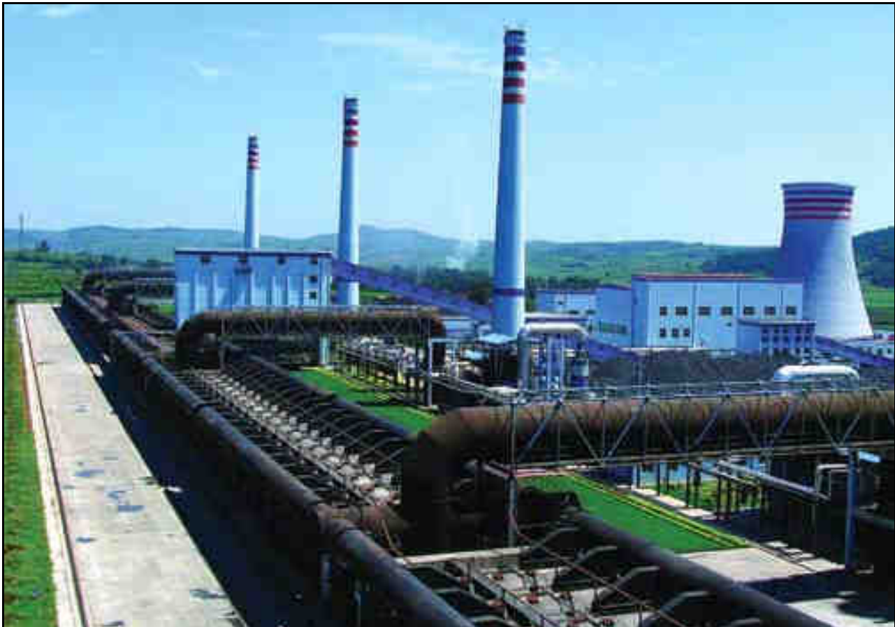
Figure 1.8: Coke Processing Plant with Associated Electricity Co-generation Plant (Courtesy SPCDI).
