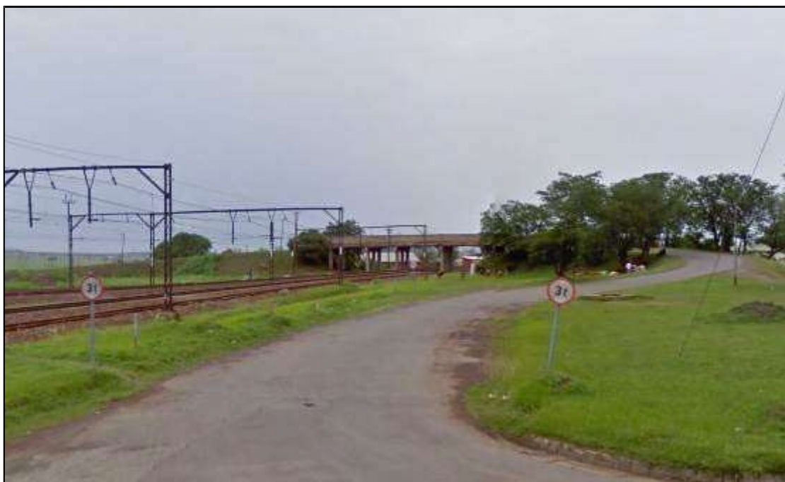
Figure 5-48: Weight Restriction on railway bridge in Colenso
