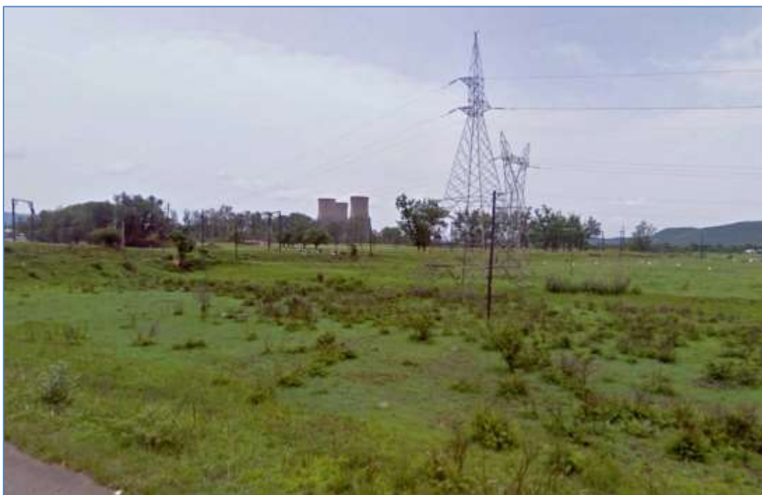
Figure 2-2: Power lines & Cooling Towers (of decommissioned Power Station)
