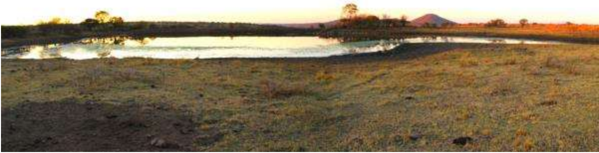
Figure 5-23: Man-made farm dam present on the proposed site
