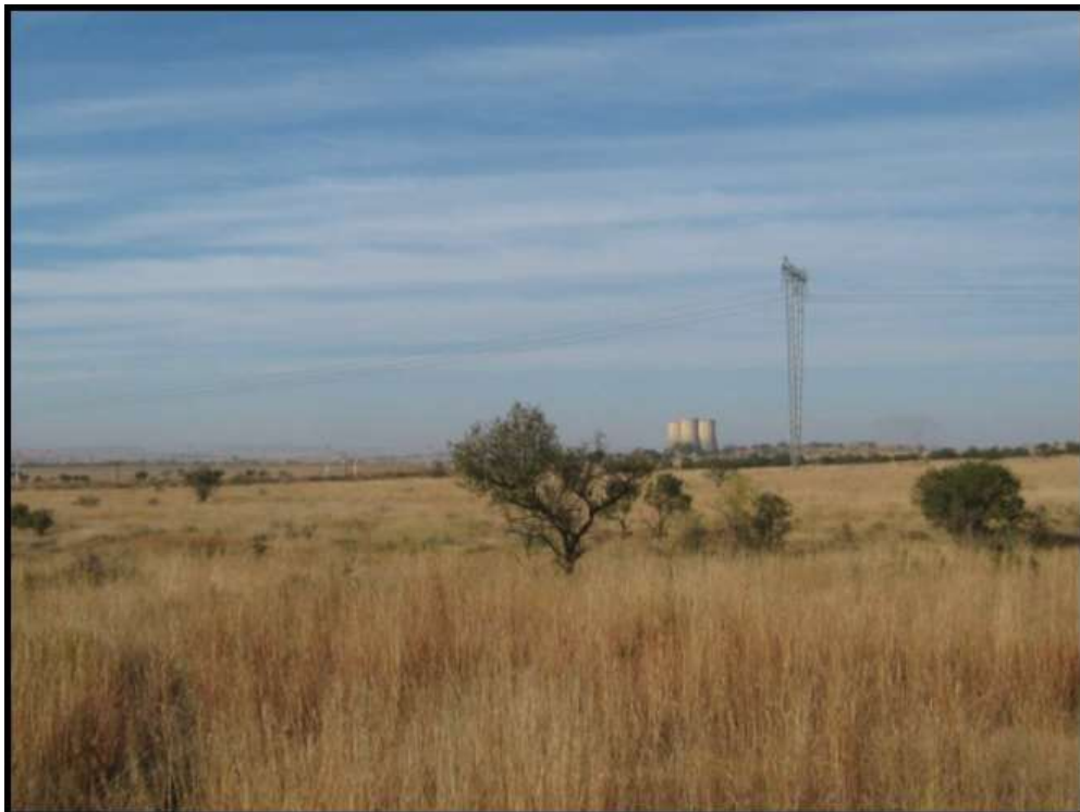
Figure 5-47: View north of Colenso showing the high voltage power lines, railway line and decommissioned cooling towers
