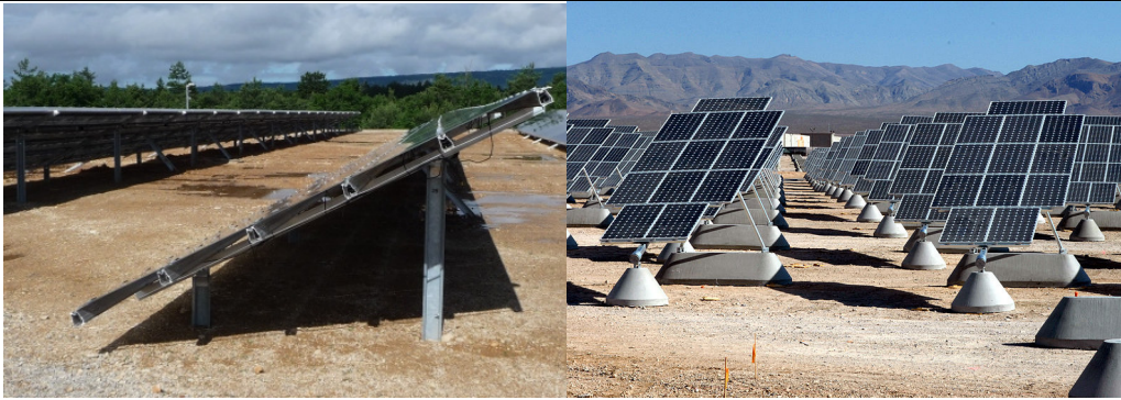
Figure 1: On the left hand side: Fixed Structures, On the right hand side: Rotating/ tracking system
