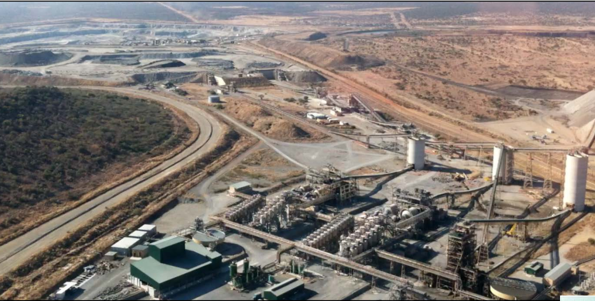
Existing PPM Plant
