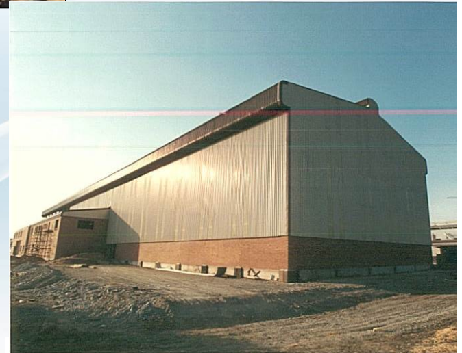
Base metal refinery – the hydrometallurgical plant at PPM will be a similar installation
