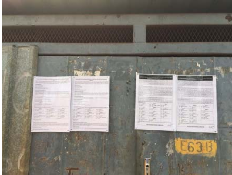
Water Pump - Magalane
