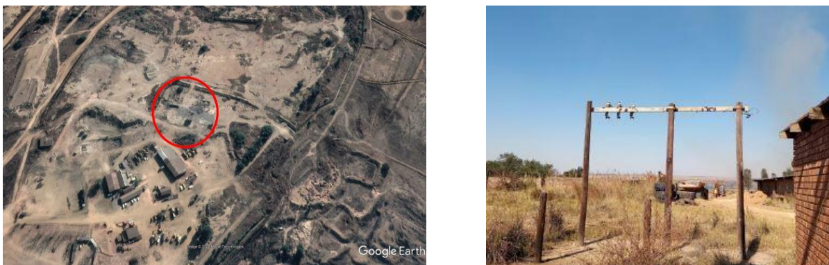
Figure 8: Decommissioned Eskom Supply Point on the proposed site
