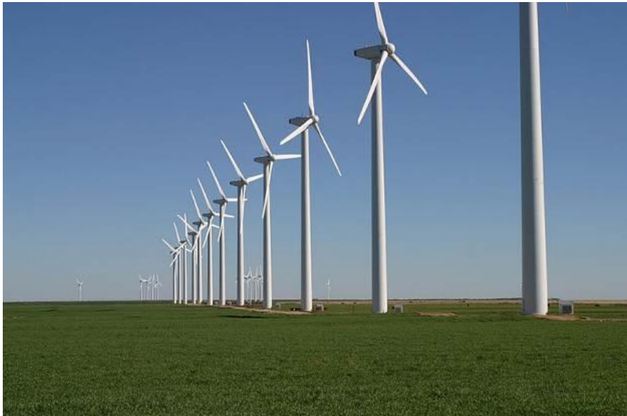
Figure 1: Brazos Wind Ranch located in Texas, USA 1
