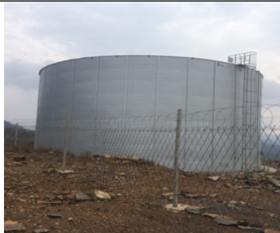
RESERVIOR TERMINATION OF PHASE 3
