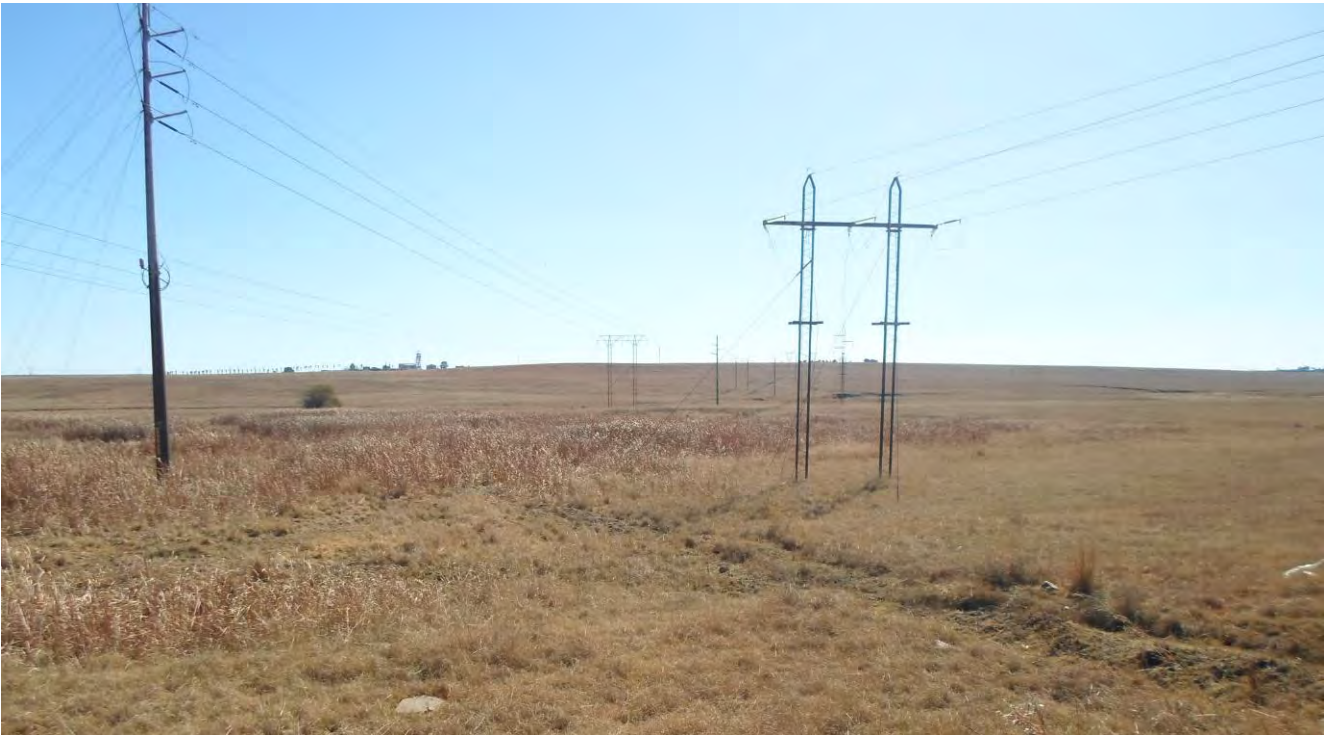
Plate 5: Photo 5: View of the proposed pipeline route along powerline servitude (Photograph © by Author 2022)
