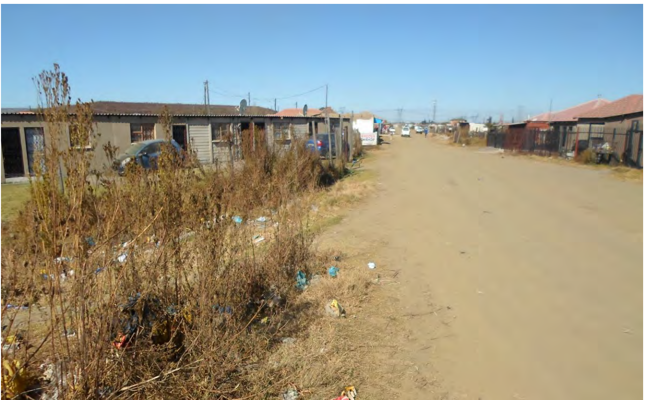
Plate 14: Photo 14: View of proposed pipeline route cutting through a built-up area (Photograph © by Author 2022).
