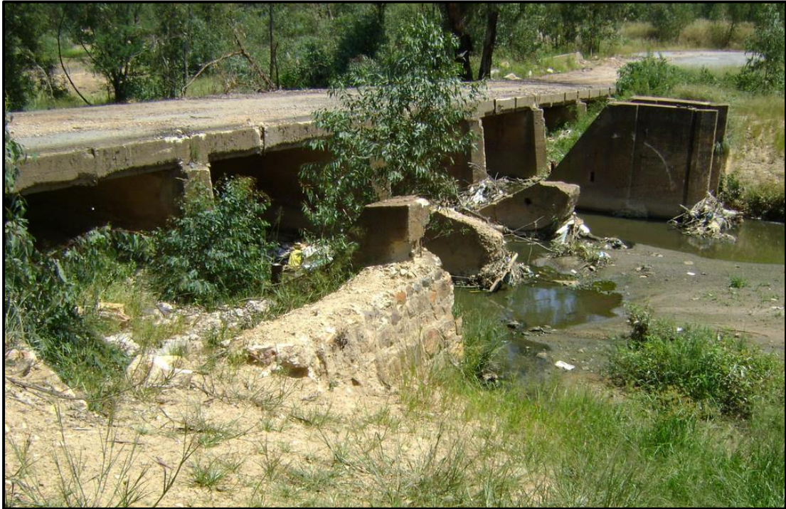
Figure 9. The older features in relation the (old) bridge
