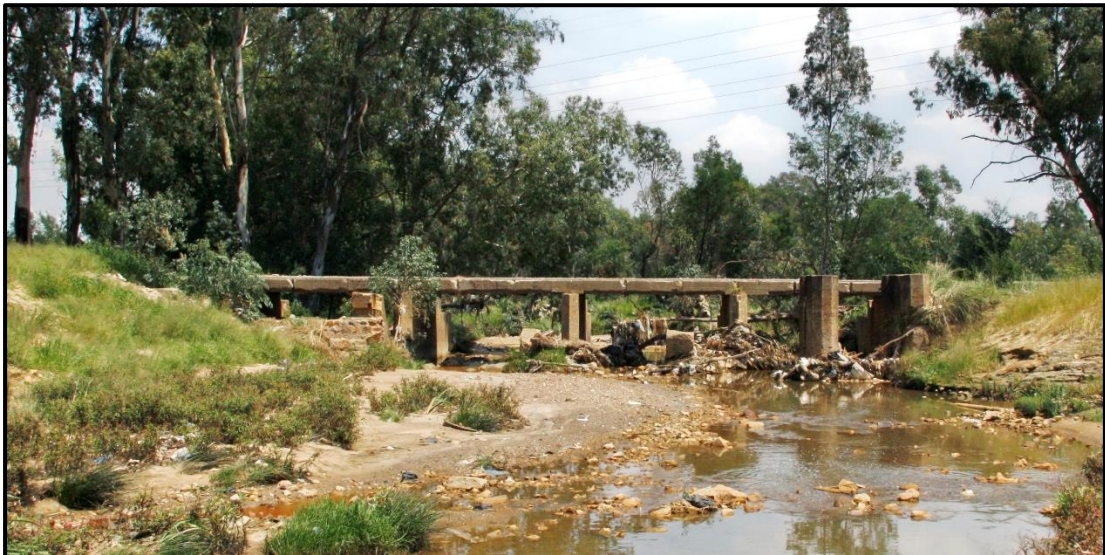
Figure 13. Side view of the old bridge, looking downstream
