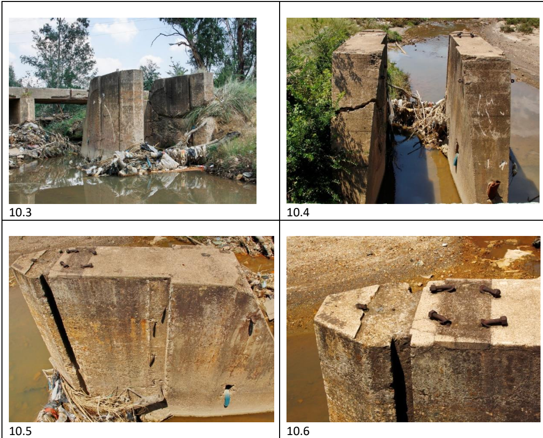
Figure 10. Details of the older features next to the bridge
