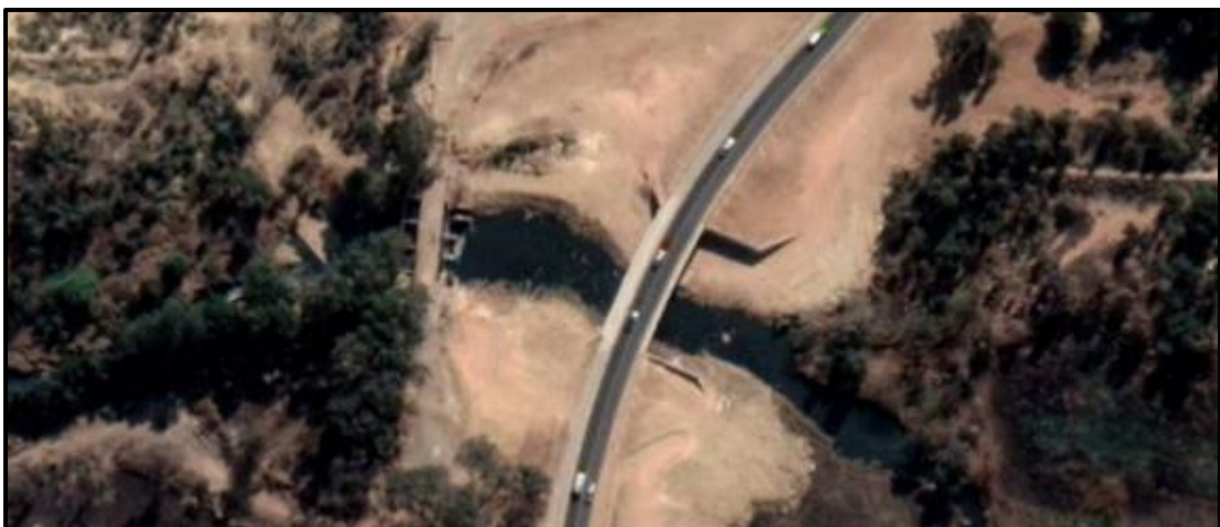
Figure 11. The old bridge on the left and new one on the right (Image: Google Earth)
