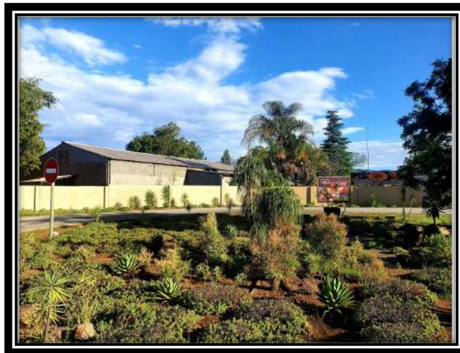
Photograph 5: Vacant Business Building
