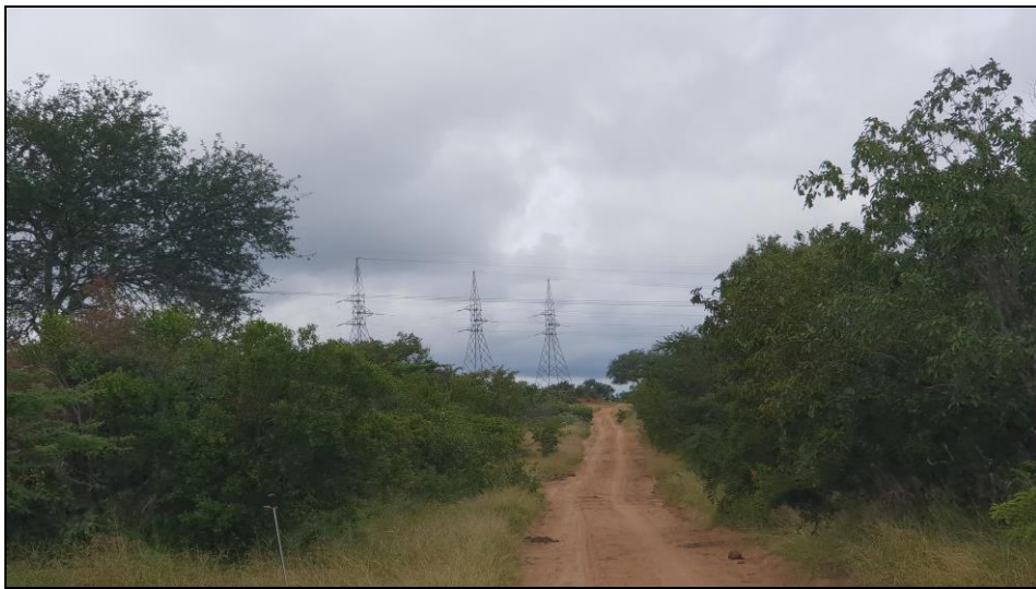
Figure 7: General view of the existing infrastructure (roads and power lines)
