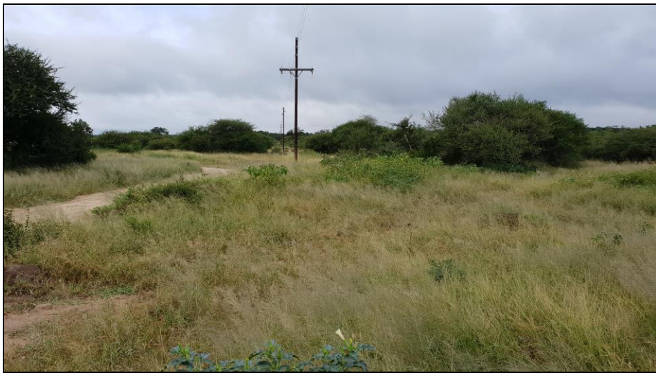
Figure 10: General view of the existing infrastructure (roads and power lines)
