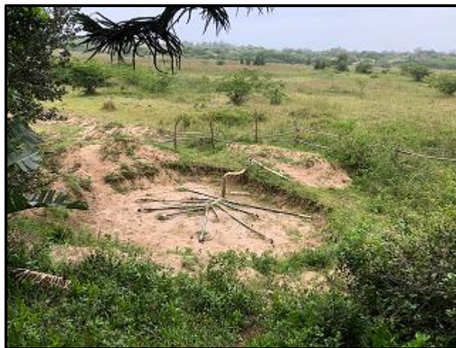
PLATE 3: WELL POINT SYSTEM WITH POOL PUMP
