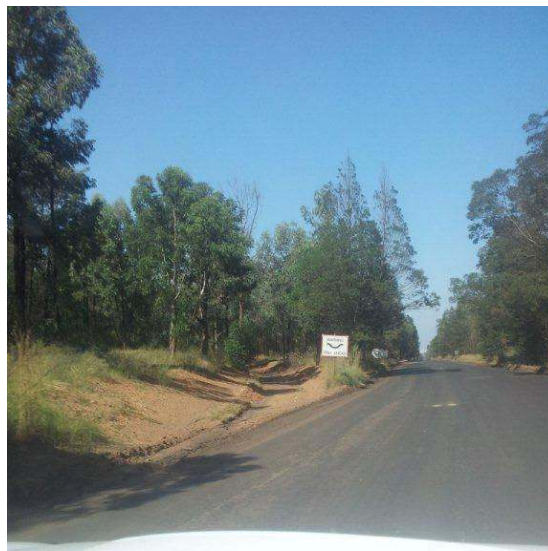
Figure 3.7: Access and on-site haul road examples of surfacing to reduce dust (from a mine previously operated by the applicant in Mpumalanga).
