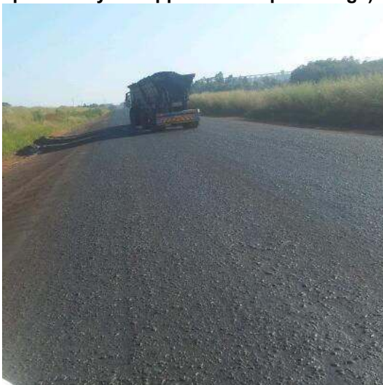
Figure 3.7: Access and on-site haul road examples of surfacing to reduce dust (from a mine previously operated by the applicant in Mpumalanga).
