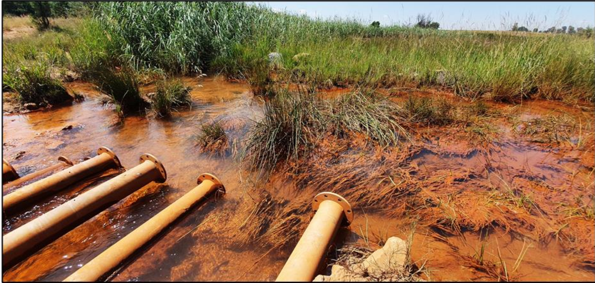
Figure 8-3 Yellow boy associated with Acid Mine Drainage (T2 – March 2020)
