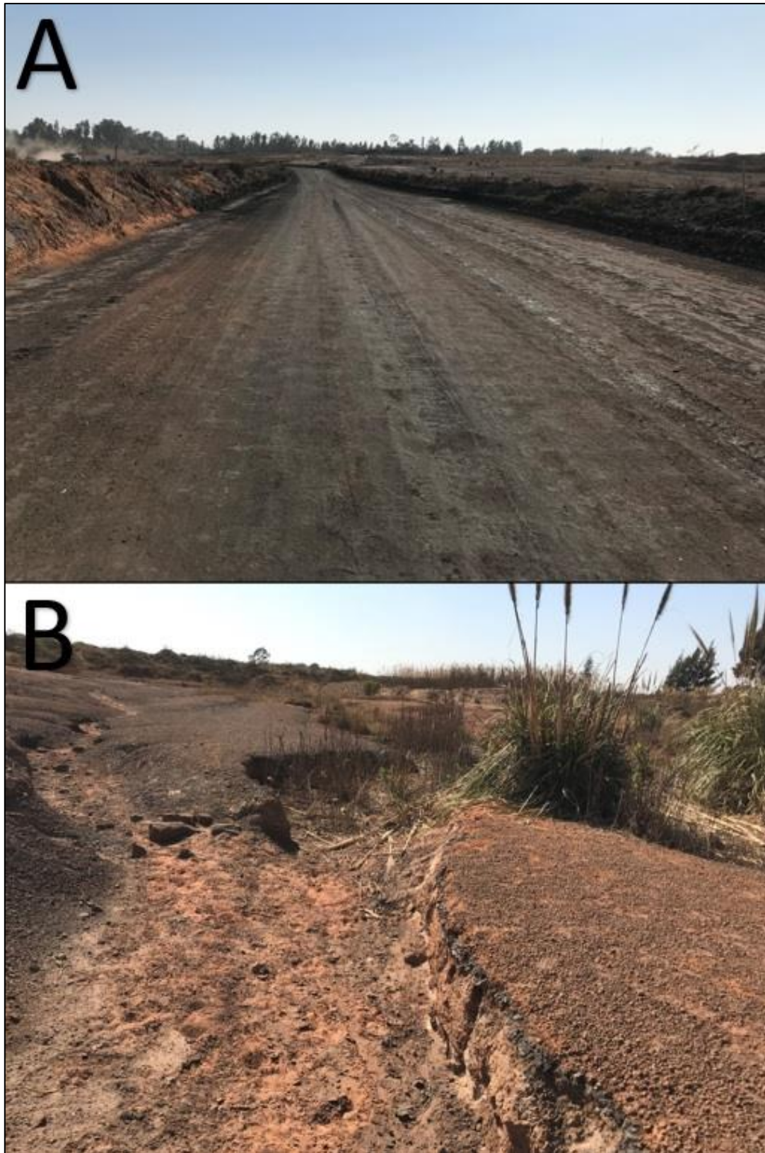
Figure 8-13 Components contributing to an increase of water inputs within delineated wetlands. A: Artificial surfaces within close proximity to HGM 1. B: Drainage lines/gullies within the wetland's catchments
