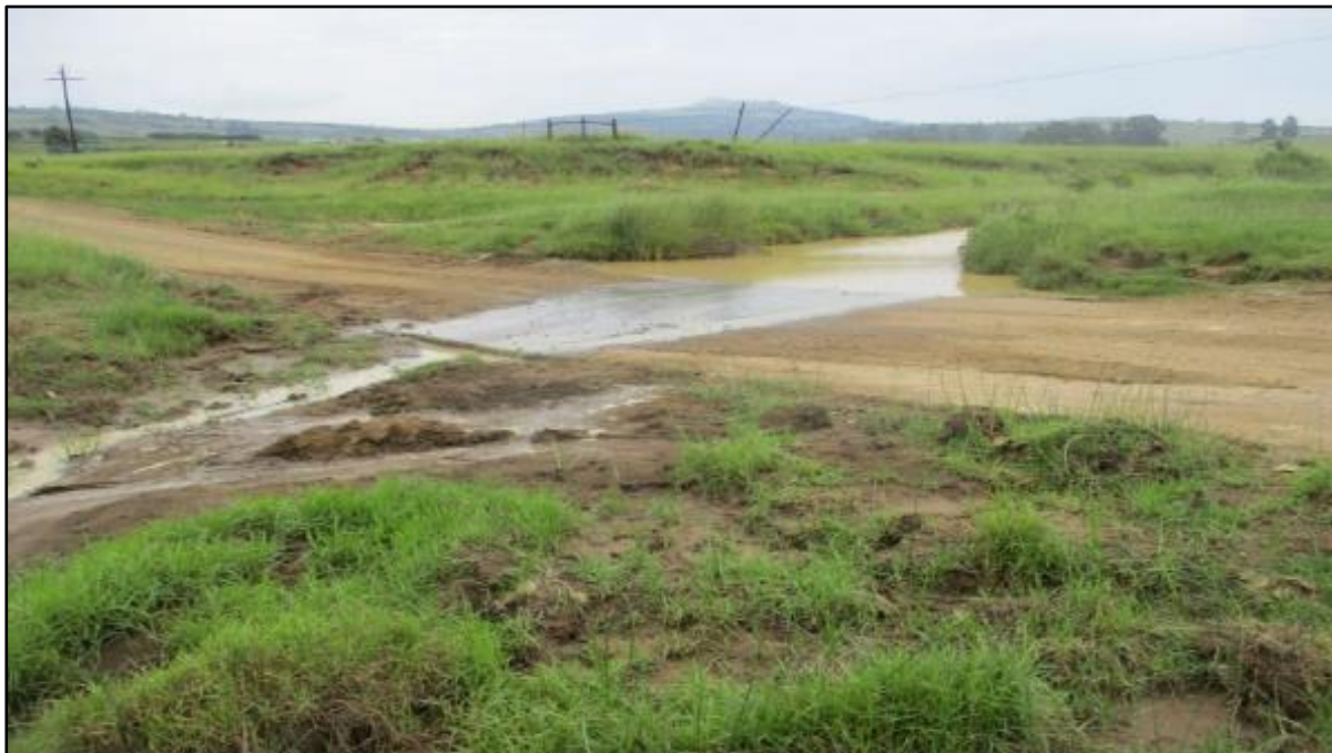
Photo 4: Showing View of crossing 4 with short to medium grasses and reeds adjacent to road and Stream.
