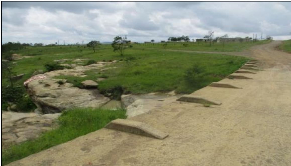
Photo 2: Showing upstream view from crossing 2 with tributary flowing towards the culvert
