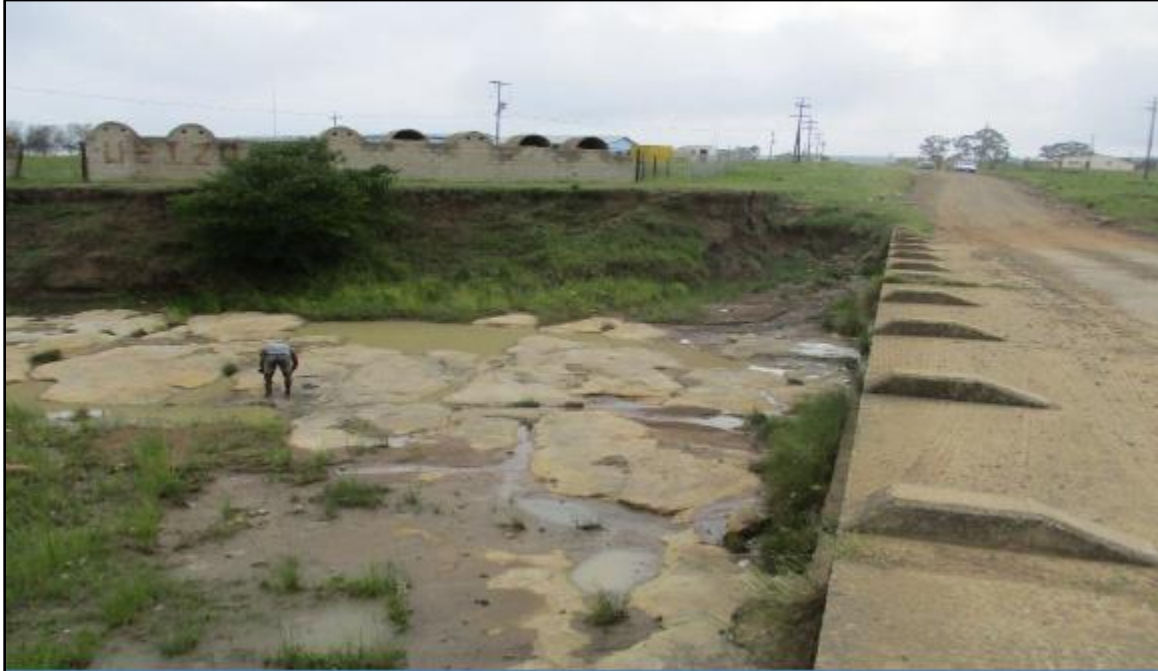
Photo 1: Showing sandstone outcrops on downstream section at watercourse 1.
