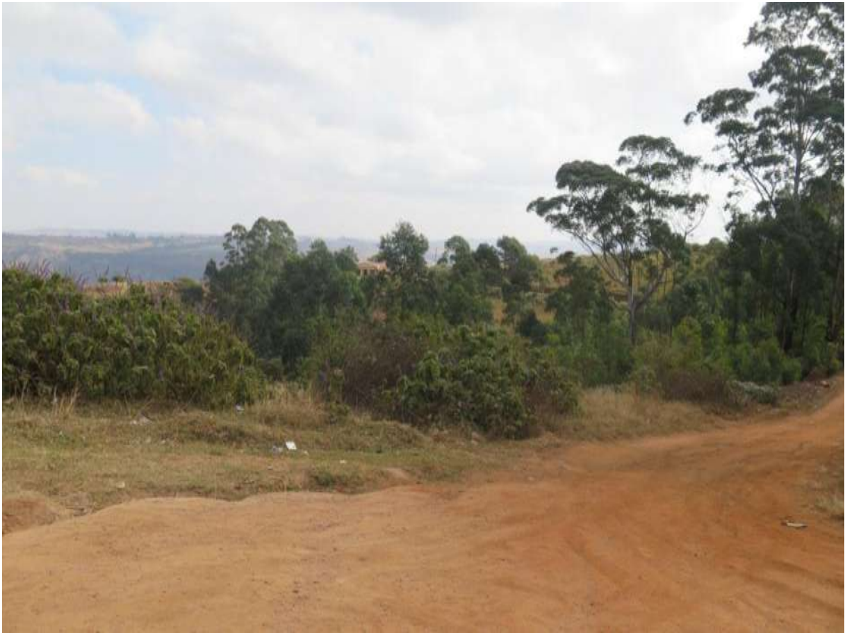
Photo 7: Erosion and alien plants next to road in the more "built-up" section.
