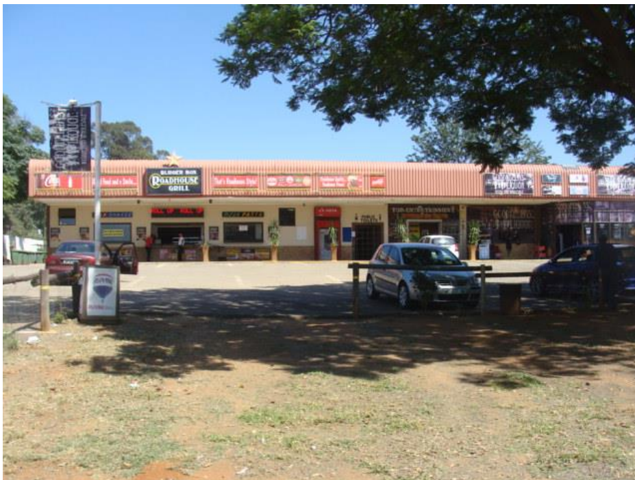
Figure 7: View of a commercial infrastructure.
