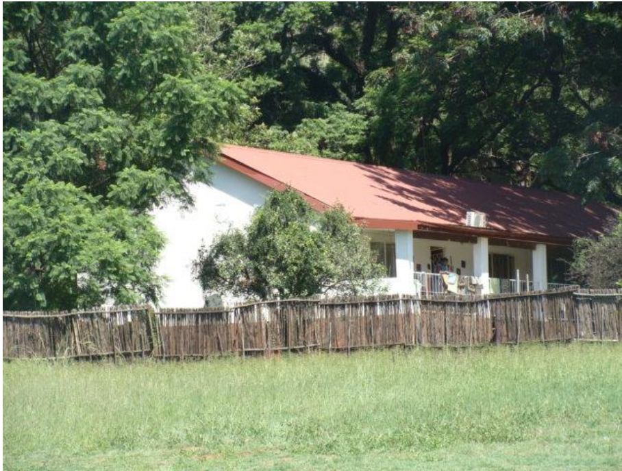
Figure 15: Another residential building older than 60 years.
